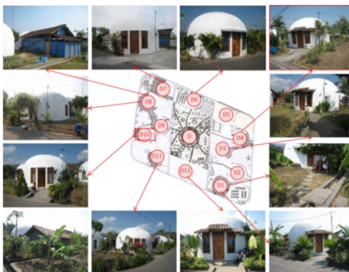
Figure 11. Existing block D
