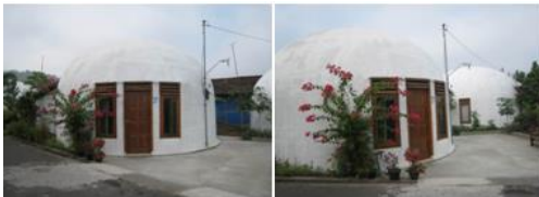
Figure 17. Conflicts access due to the use of rigid pavements
